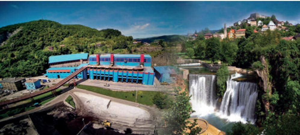
bosna is active in production since 2004 and equipped with 3 SAF and of 26 MW total installed power produces around 18.000 tons yearly.
