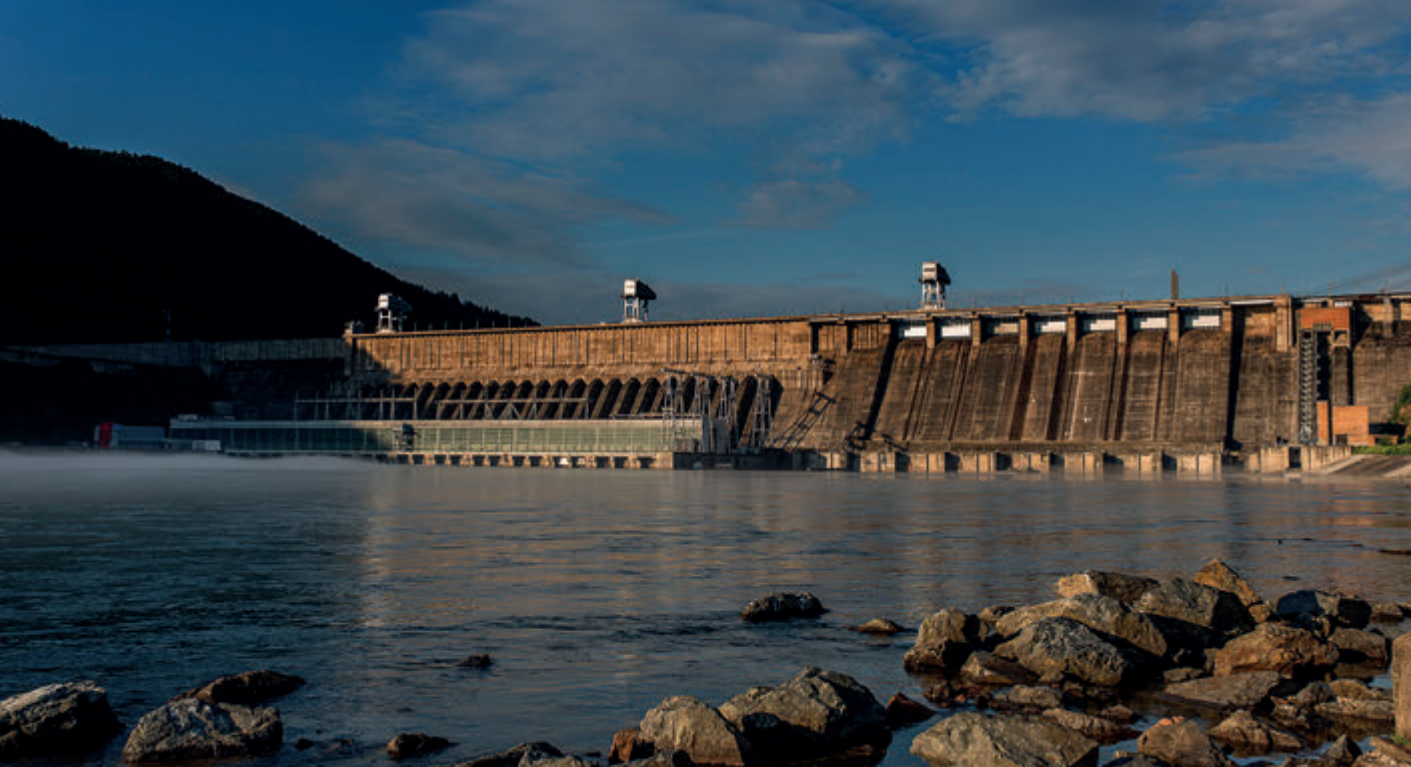
Rusal's massive energy and metals complex on the Angara River in the Krasnoyarsk region (Central Siberia)
