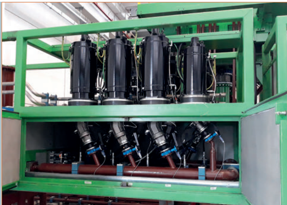
PE. Energy Saving System, assembly vertical pumps (detail) PE. Energy Saving System con pompe montate verticalmente (dettaglio)
